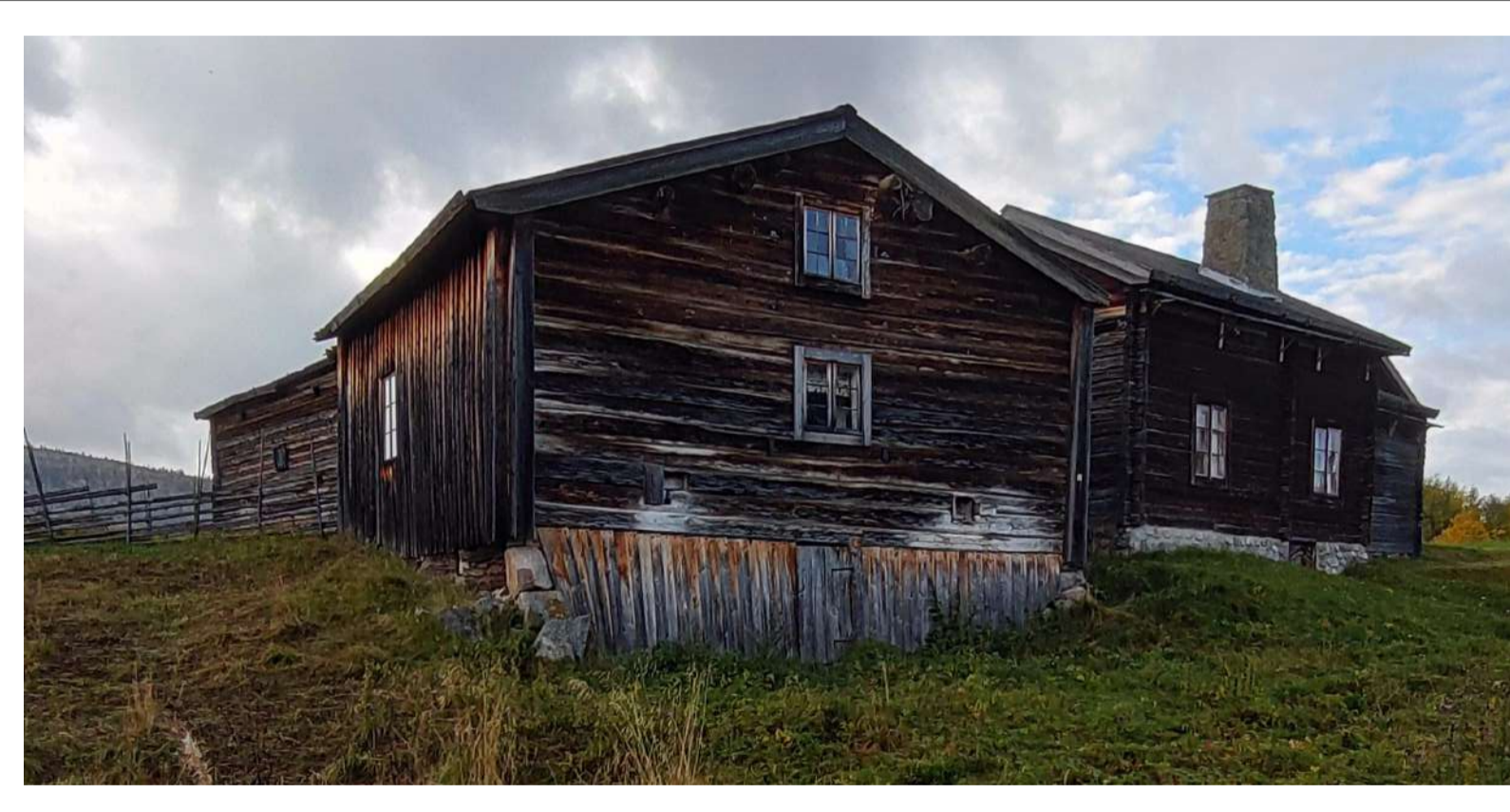
RAISED FOUNDATION CLAD WITH PLANKS
