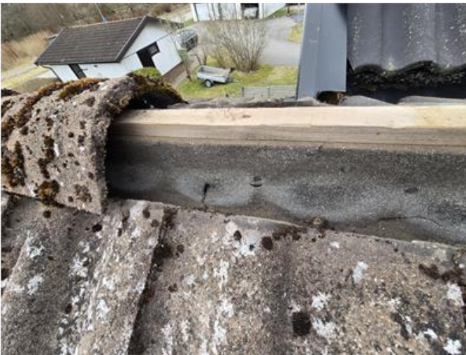
Tak: Otätheter i underlagspapp undernockpannor.
