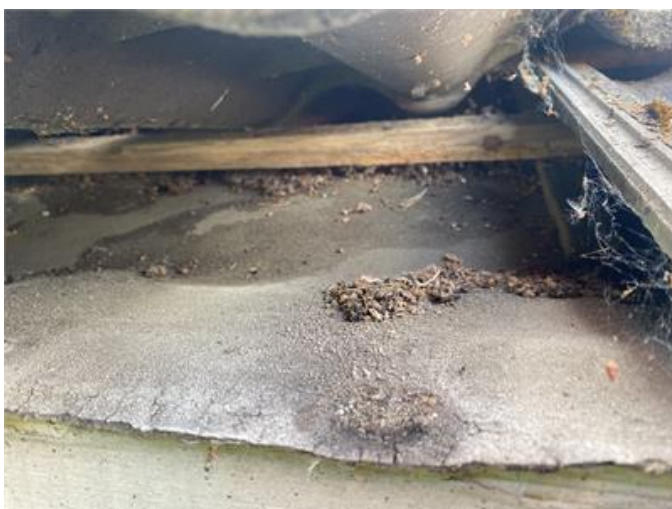
Yttertak under pannor
