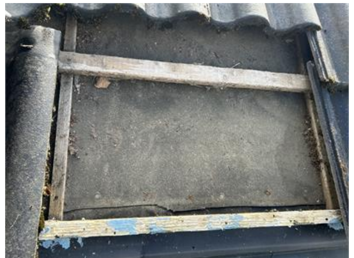
Garage tak: Stickkontroll under pannor torr papp noteras.
