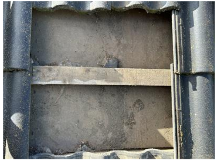
Tak: Stickkontroll under pannor.
